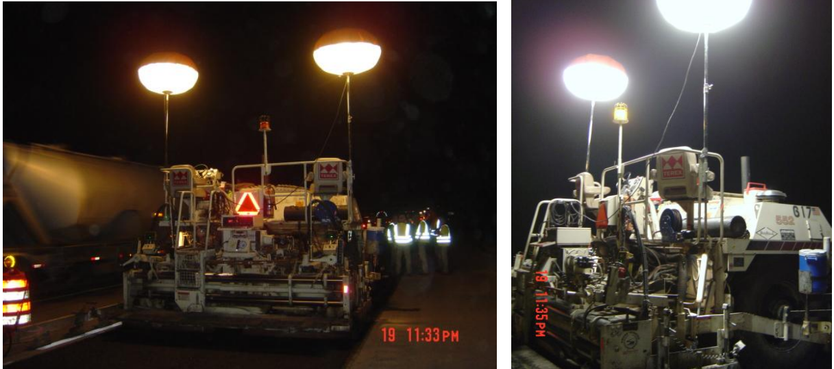
Figure 2.9 Balloon Lights in Highway Projects
