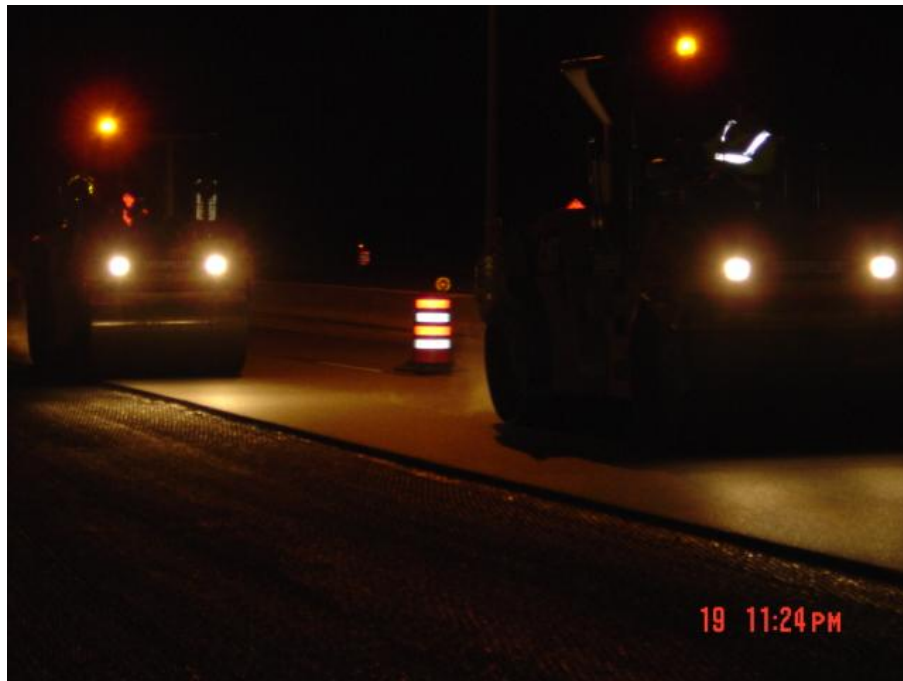
Figure 3.19 Headlights for Roller (I-74)
