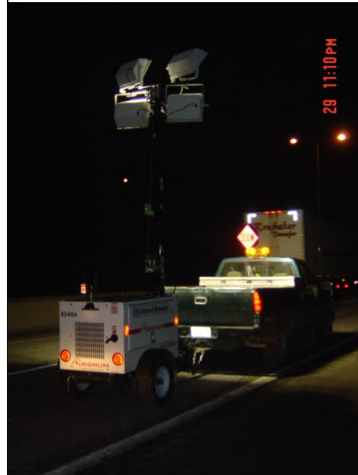
Figure 3.20 Light Tower to Illuminate Flagger Station (I-74)
