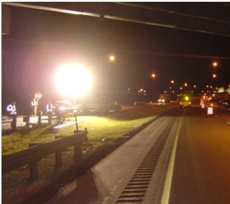
Figure 4.45 Girders Repair Activity
