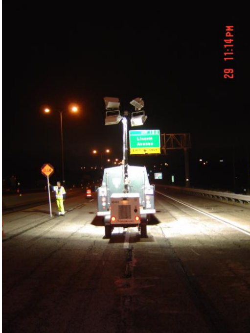
Figure 3.20 Light Tower to Illuminate Flagger Station (I-74)
