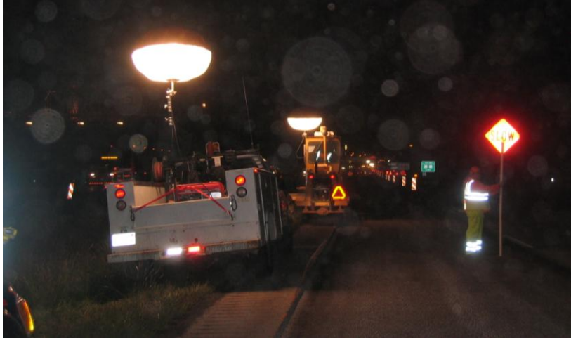
Figure 3.15 Balloon Light to Illuminate Flagger (I-70)
