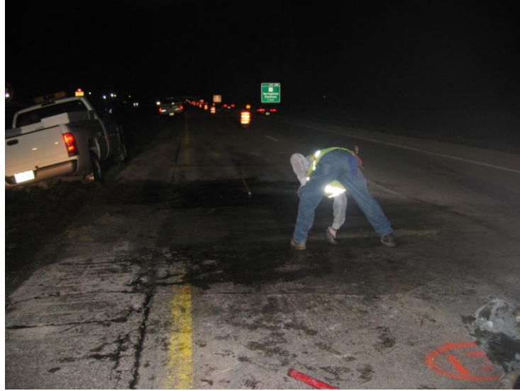
Figure 3.11 Patching Operations (I-72)
