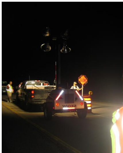
Figure 3.12 Light Tower to Illuminate Flagger Station (I-72)
