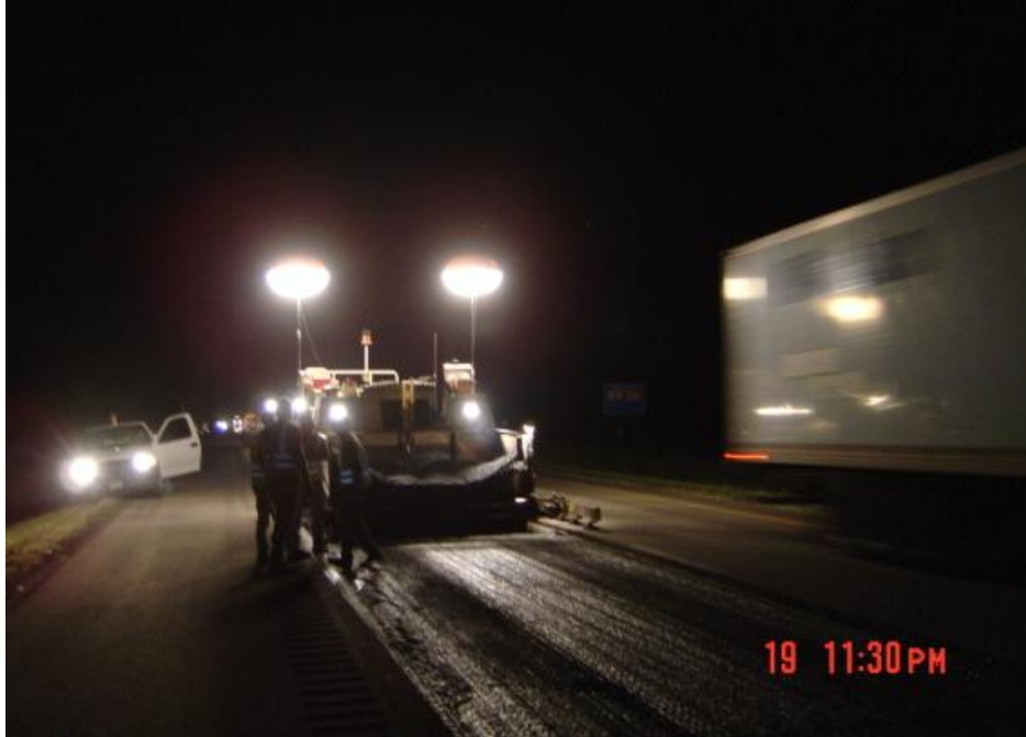
Figure 4.35 Pavement Equipment Using Two Balloon Lights
