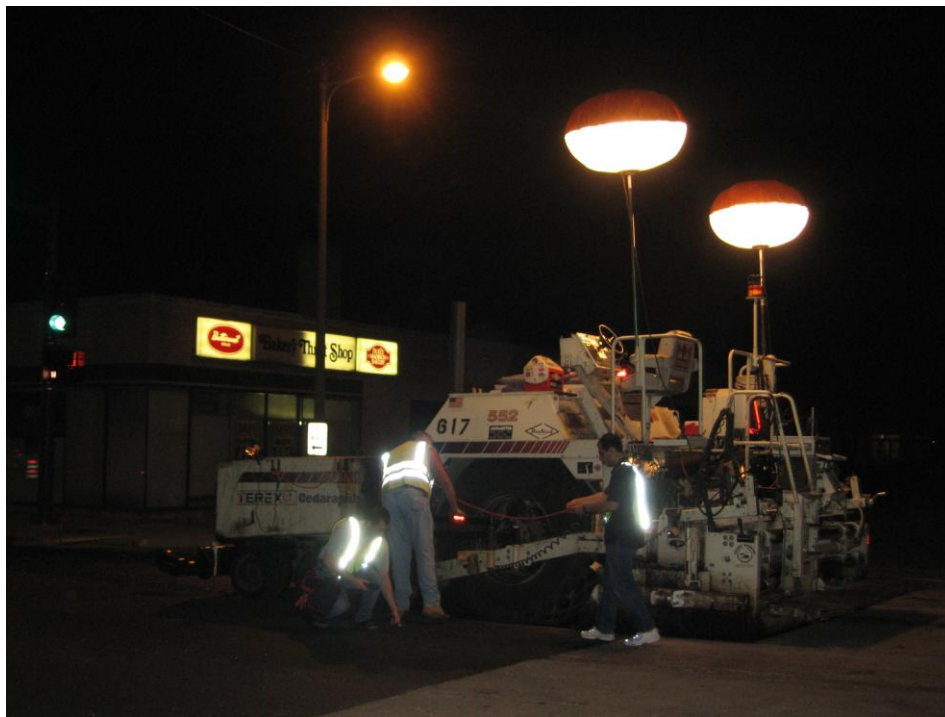
Figure 3.8 Balloon Lights on Paver (IL-23)
