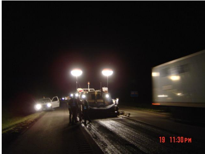
Figure 3.1 Balloon Lights on Paver (I-80)
