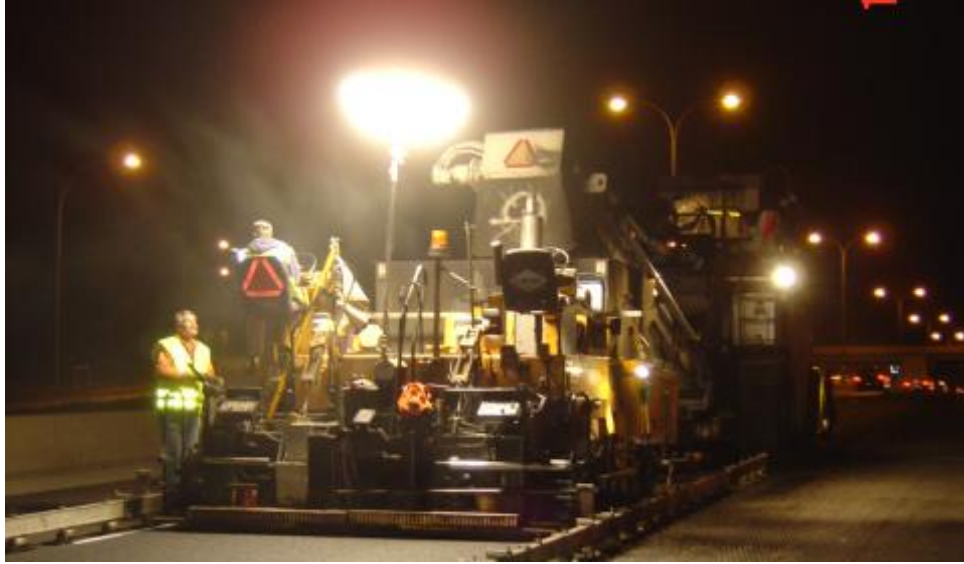
Figure 4.26 Paving Bituminous Surfaces Activity
