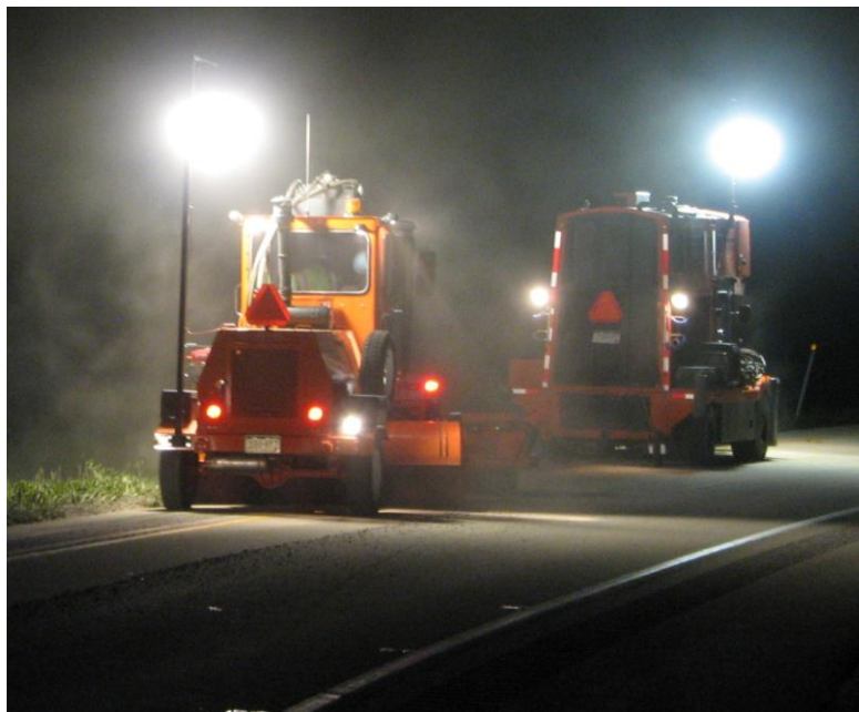
Figure 4.64 Pavement Cleaning and Sweeping Activity
