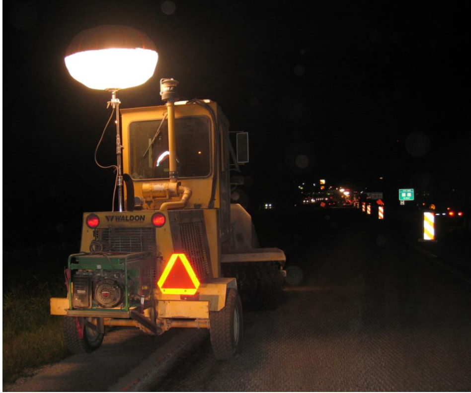
Figure 4.28 Pavement Cleaning and Sweeping Activity
