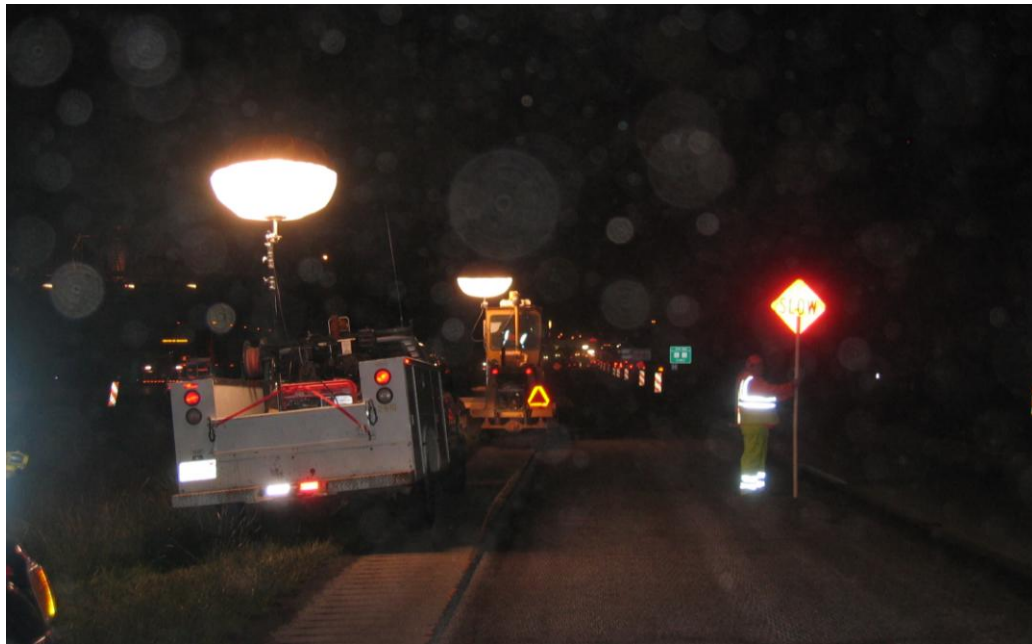
Figure 4.29 Work Zone Flagger Station
