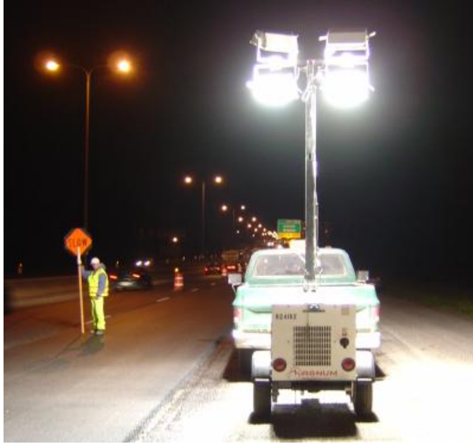
Figure 4.47 Work Zone Flagger Station
